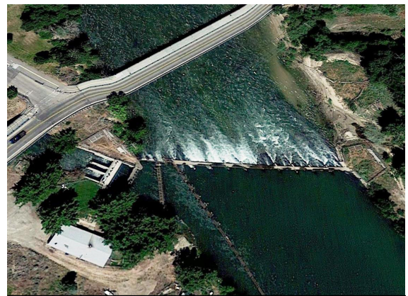
The Nampa & Meridian Irrigation District diversion on the Boise River near Barber Park.
