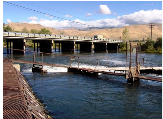
The Ridenbaugh Canal headgate on the Boise River near Barber Park. (NMID Photo)
